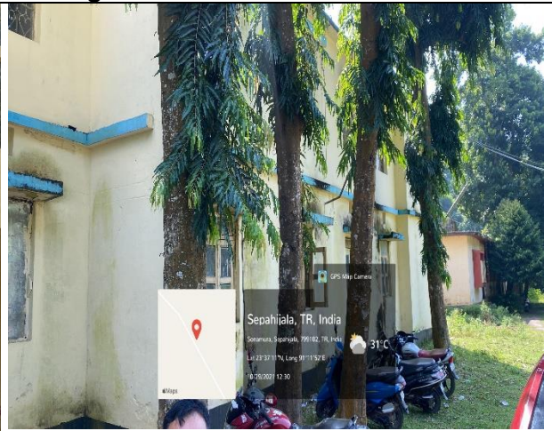
Looking from north to south, showing the GTDL building to be demolished and the small office behind also marked for demolition
