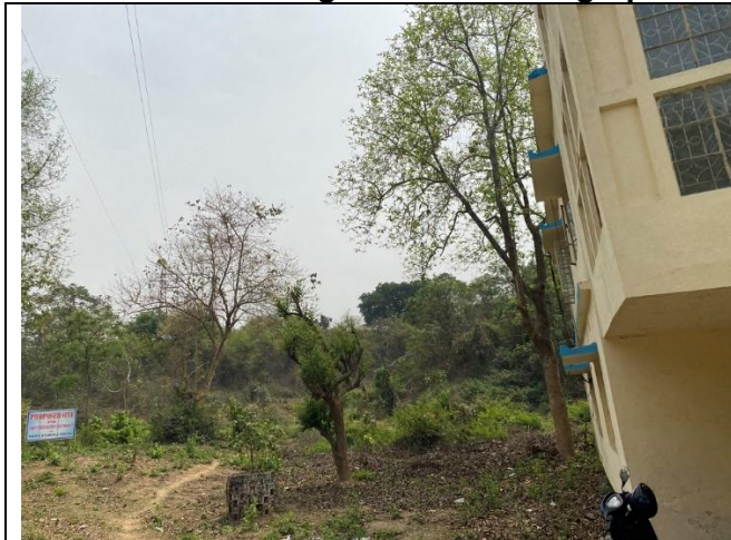
Looking from GTDL building (south) to be demolished into north (HRSG site)
