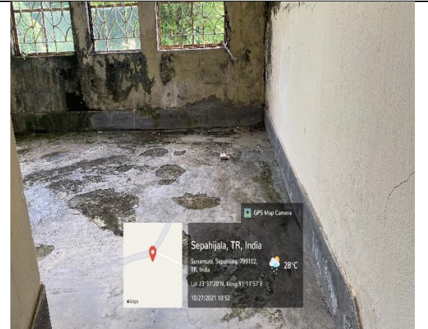
GTDL building inside
