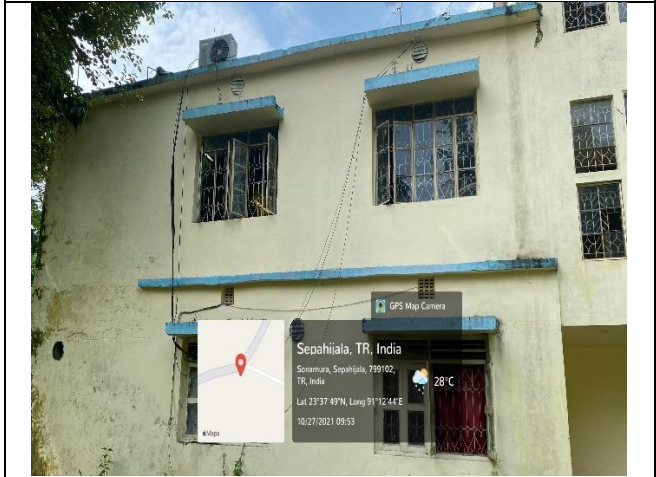
GTDL building marked for demolition – external view
