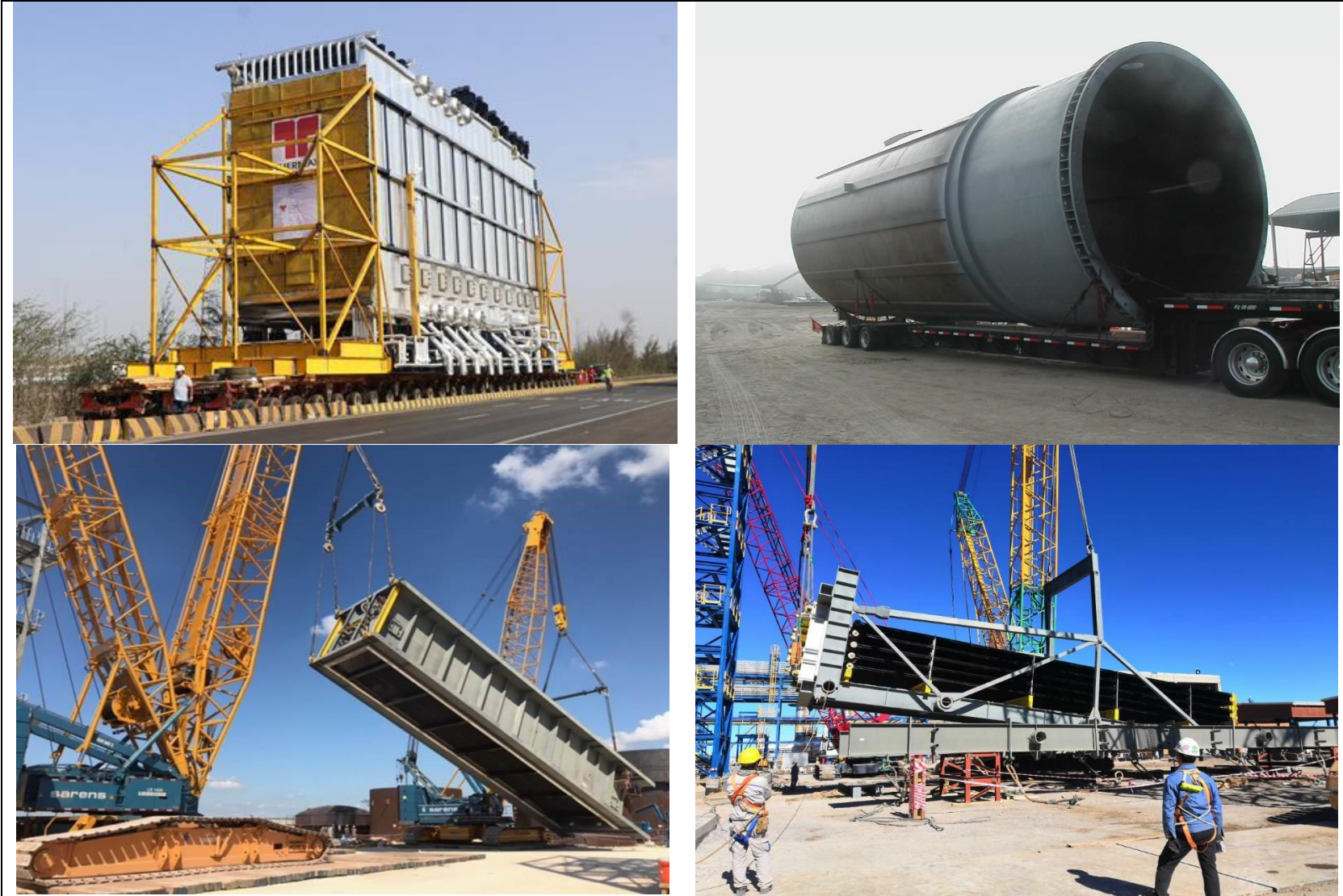
Figure 2-13: Representative Images of Transport and Assembly of CCGPP Oversized Modules
